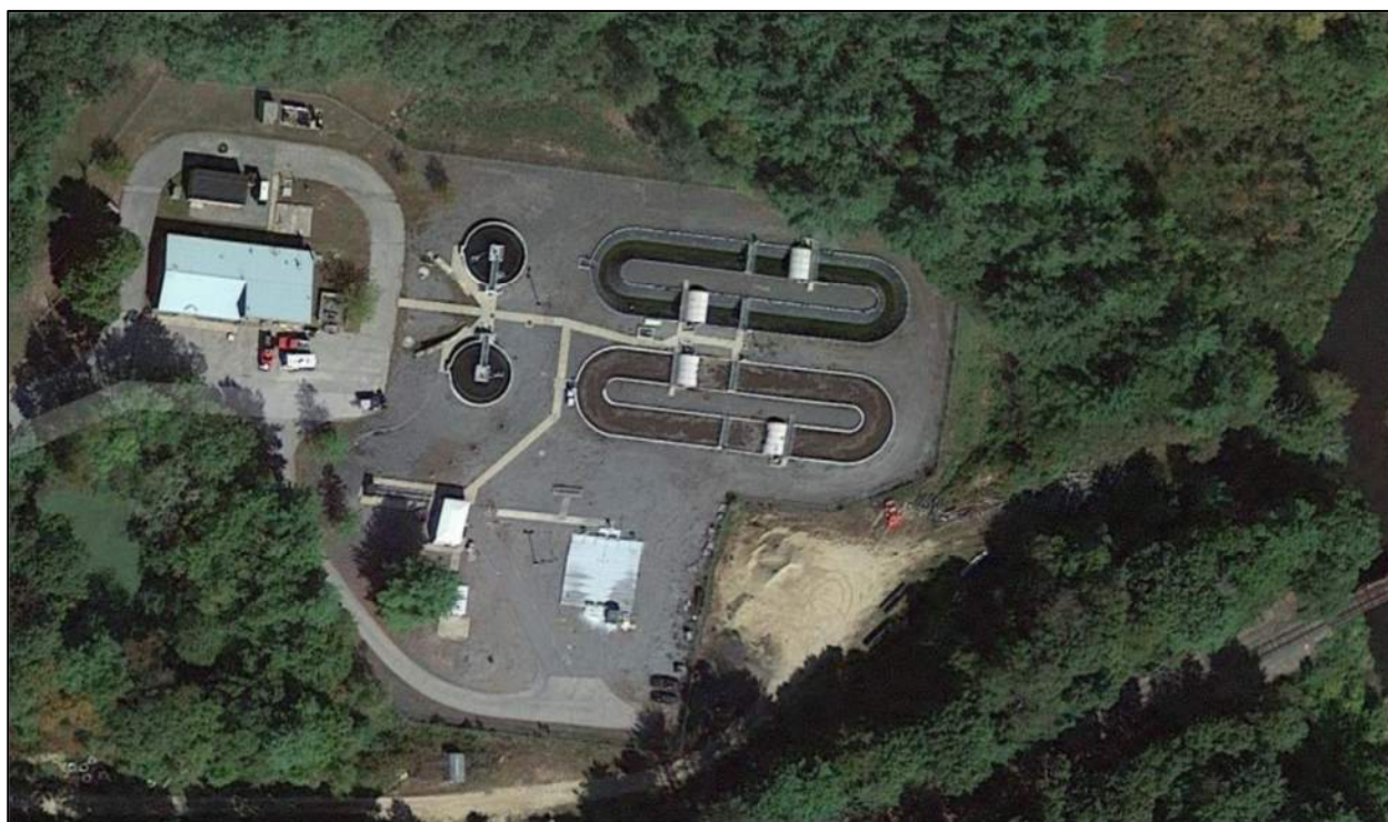
Figure 2-1: Existing Barre WWTF Aerial
